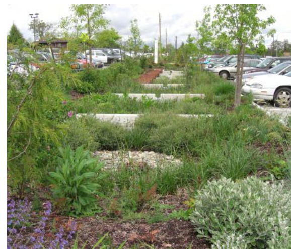
Storm water retention areas within a parking lot
