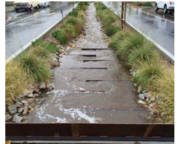
Median right-of-way bioswale
