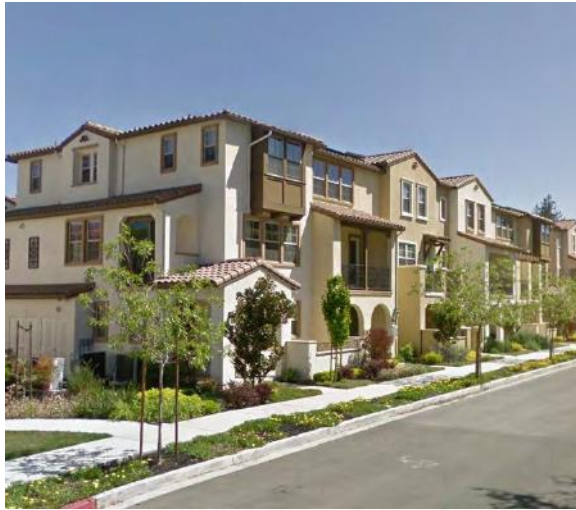
New traditional Spanish-style neighborhood with articulated façades and entries.
