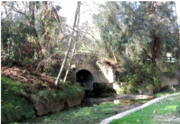
Stone-faced concrete arch bridge supporting bridle path at Lemon Creek. View looking north.
