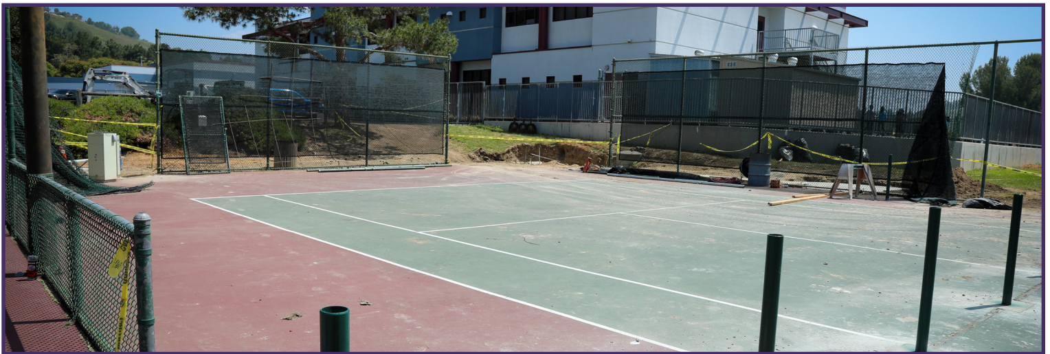
Court A at Walnut Ranch Park Under Construction
